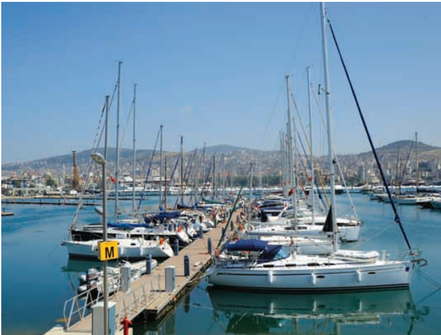
Marinturk Istanbul Cityport has specific types of piers for different sizes of vessels.
