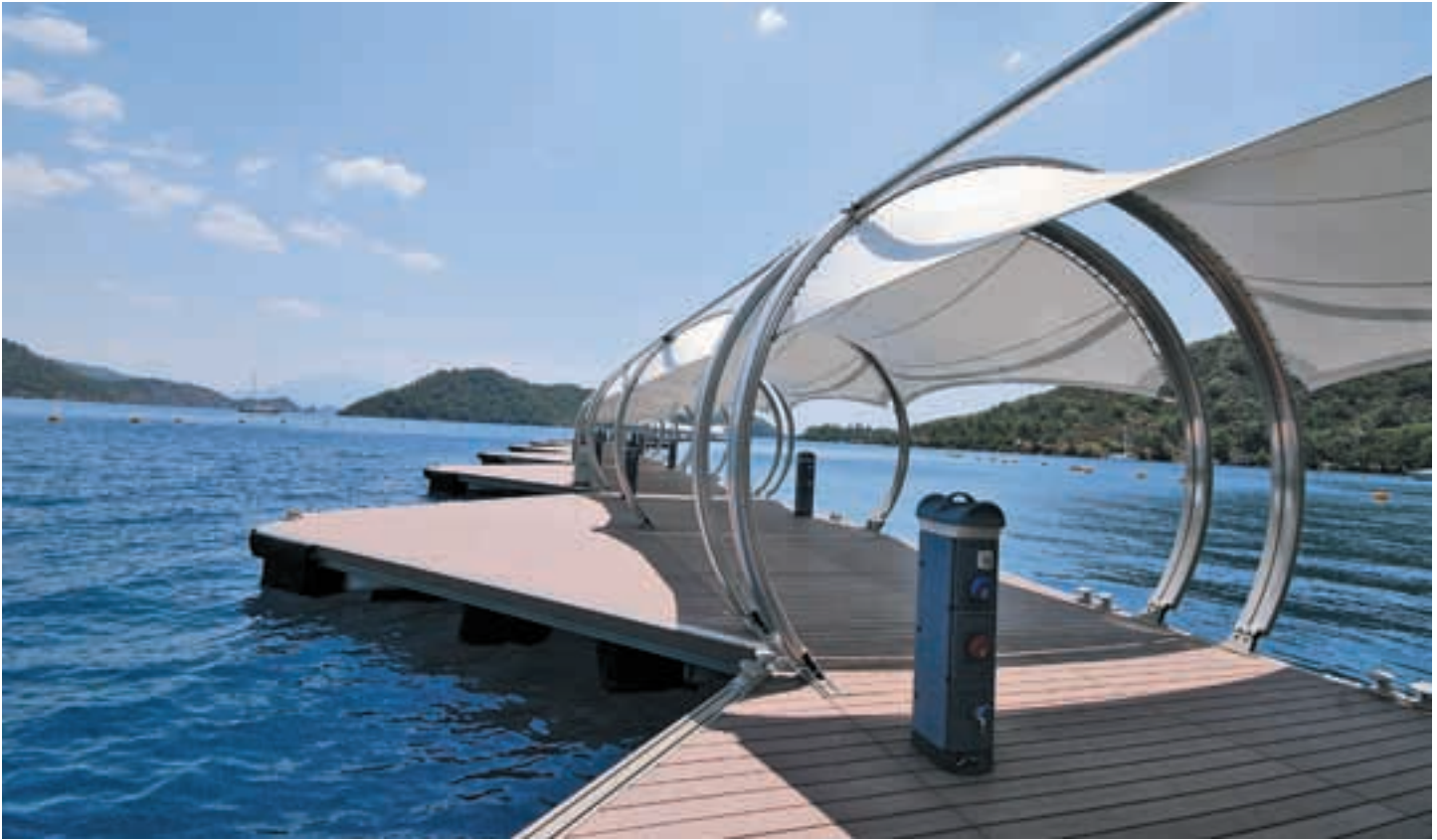
The tented pier provides a cool shade from the hot summer sun
